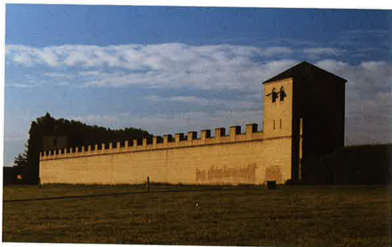
Right: Another view of the partially reconstructed tower and walls at Xanten on the Rhine. This shows how towers under the Principate did not protrude and how the walls did not have deep moats in front, being designed merely to break the impact of attack.
